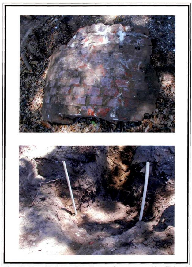
Figure 12. Views of the former well. Top: Fragment of masonry recovered from fill above the well. Bottom: Intact brick lining exposed by backhoe excavations.
