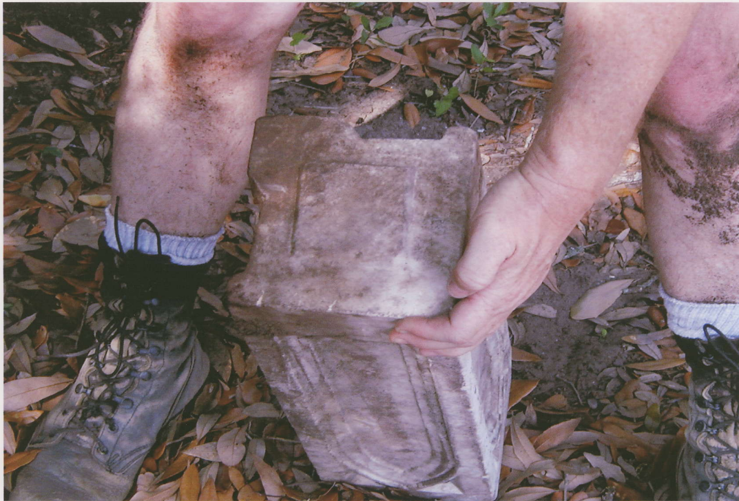
Tenon on base of corner post.
