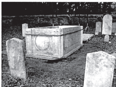
The now-together sides and corners are held with a strap until set.
