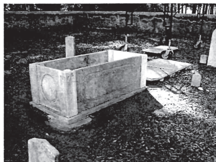
Straps removed and corner foundation repaired, the crypt is free standing.
