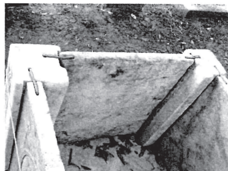
The cramps securing the corners to the sides and end of the crypt.
