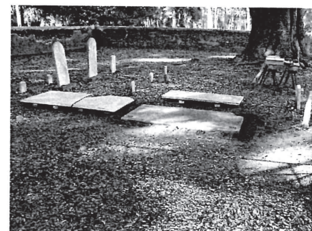
Top - portable hoist Lower - marker removed from foundation
