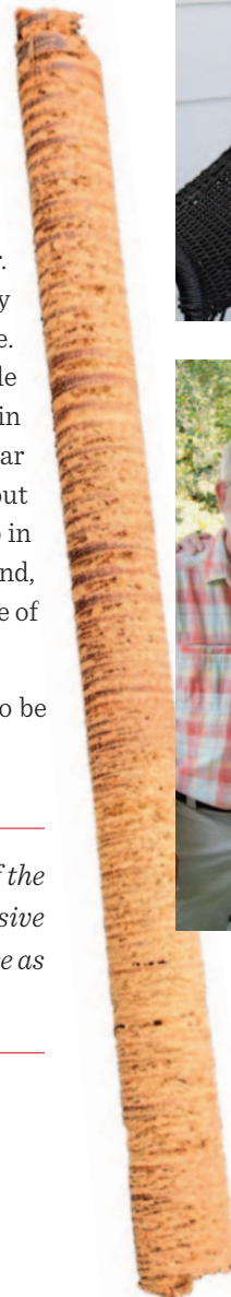
CORE SAMPLE FROM AN ORIGINAL RAFTER IN THE HEXT HOUSE
