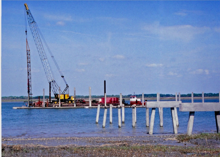
Marina under construction - 1989
