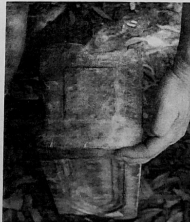
Tenon on base of corner post.
