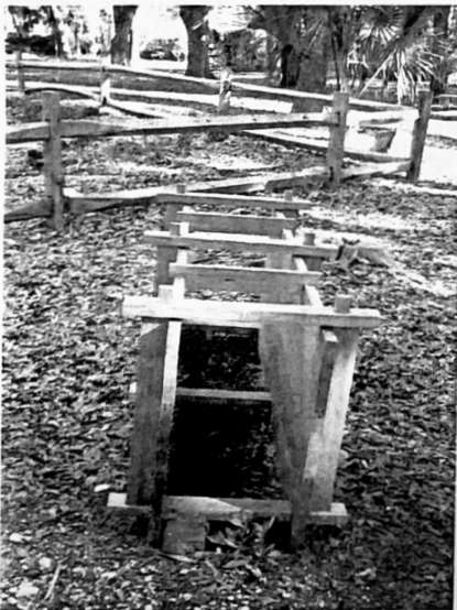
Cradle parts were not attached so they could be removed easily and reassembled for the next section.
