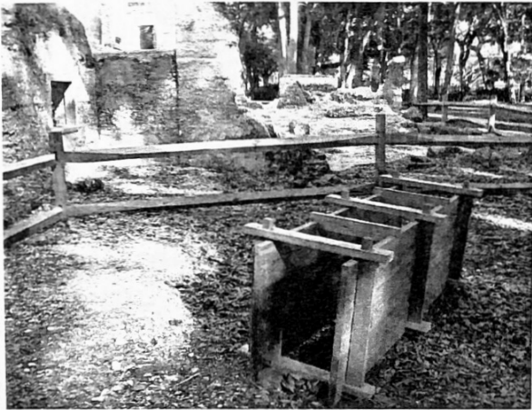
Cradle parts were not attached so they could be removed easily and reassembled for the next section.
